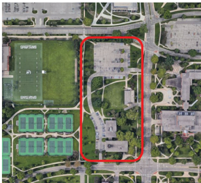
Aerial photo site location.
